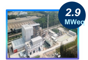
Industrial Waste to Energy
