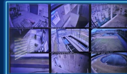
Example of the screen at Unified Operation Center (UOC)
